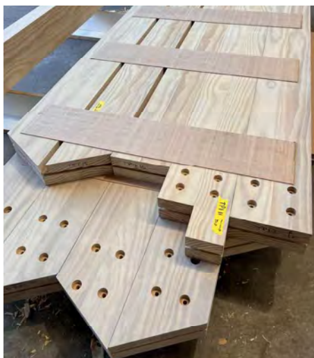
Above: Fabricated beams, ready for installation.
