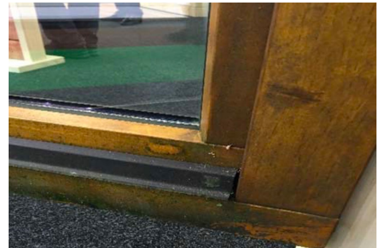
No coating degradation visible
