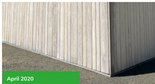
CLADDING PROJECT, NORTH AMERICA
