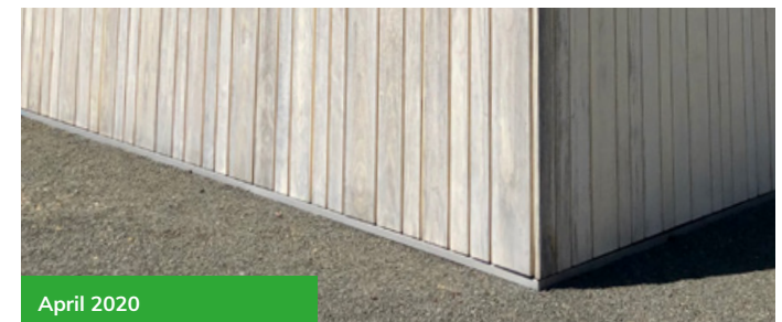
CLADDING PROJECT, NORTH AMERICA
